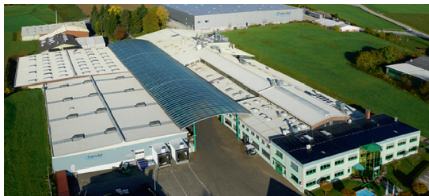
Frankenmarkt plant Austria
